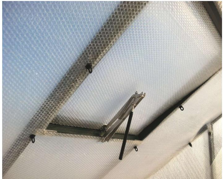
**TIP:** *Our bubble insulation can be left up year round, but if you will not be using the greenhouse during the summer, we recommend removing the bubble and storing it out of the sun. This will increase its lifespan. Bubble should only be installed on the inside of the greenhouse.*
