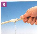
When you are done installing the mist ring, turn on the water to flush out the system BEFORE installing the mist nozzles.
