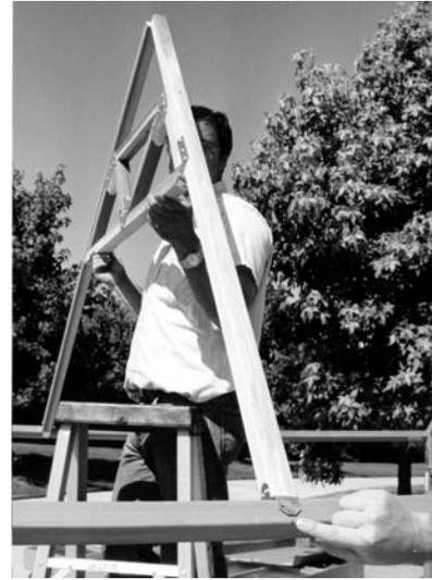
Position a roof truss at the center mark on the top plate. Align the front edge of the truss with the mark and attach it from the inside using 3/4" screws through the **untaped holes only**.
