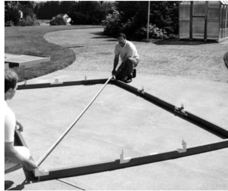
Check that the base is square by measuring from corner to corner in both diagonal directions. If the measurements are not equal, push on the longer dimension until they are equal.
