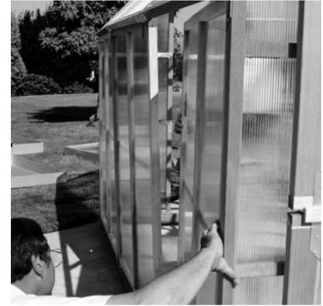
Swing the "halfway connected" second and third panels inward and press them together into alignment with the base.
