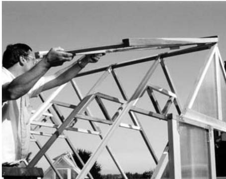
The vented side of the roof must be attached before the unvented side.
