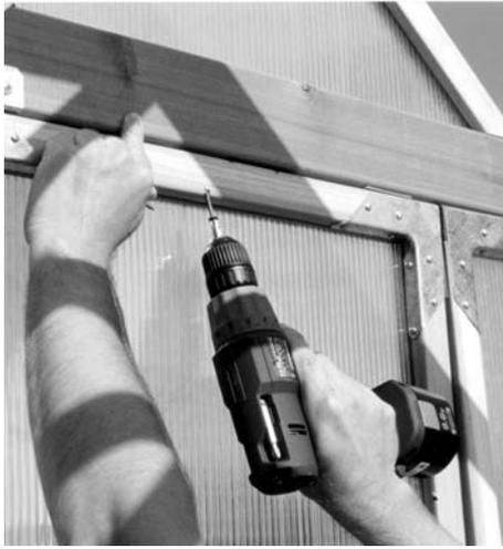
Attach the top of the panel from the inside using one 2-1/2" screw through the pre-drilled hole. See page 14 for addendum tip. Then attach the sides using four 2-1/2" screws through the pre-drilled holes.
