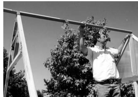
Rest the **ridge front** on to the front wall and center truss. With the ridge flush with the front wall, attach it through the connectors using 1-1/4" screws.
