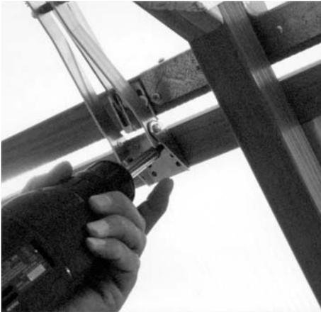
Position a vent operator near the center of a roof vent along side a truss with one bracket on the vent frame bottom and one on the adjacent roof panel blocking. Attach the two brackets using four 1-1/4" screws.
